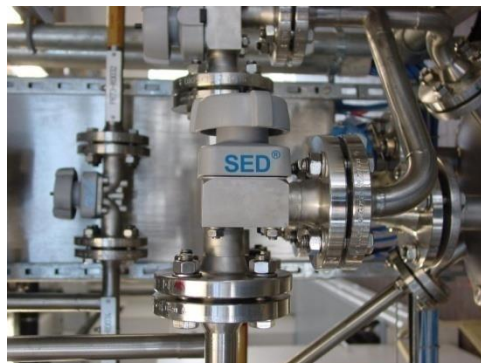
Membran- + Kugelhahn-Armaturen / Membran- + ball valves
