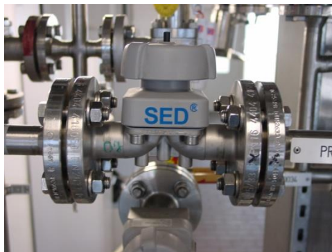
Membran- + Kugelhahn-Armaturen / Membran- + ball valves
