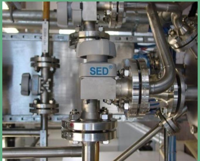
Membran- + Kugelhahn-Armaturen
